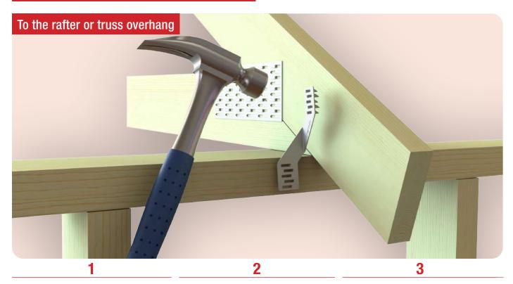
Prevent the truss or rafter from moving along the wall frame top plate by hammering a nail into the top plate, against the side, away from the Truss Tie.
